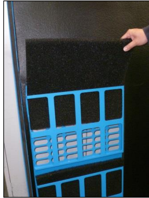
Figure 6-2 Air Pre-Filters Removal
