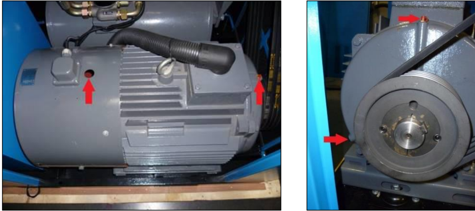
Figure 6-5 Motor Bearing Re-Greasing
