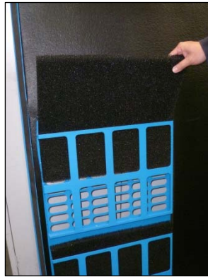
Figure 6-2 Air Pre-Filters Removal
